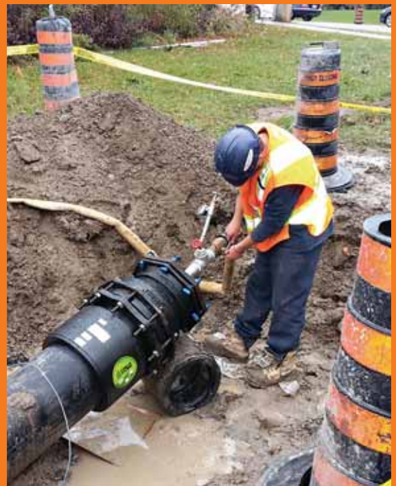
Markham, Waterworks construction, October 2013
