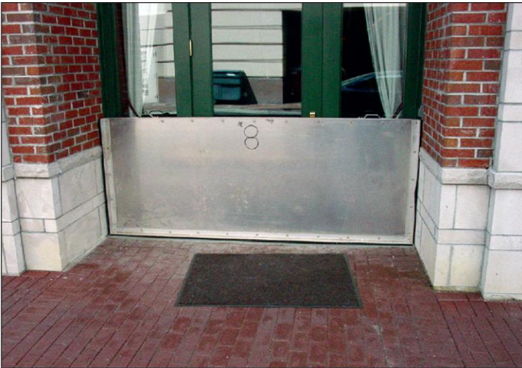
Aluminum flood shield used on exterior door
