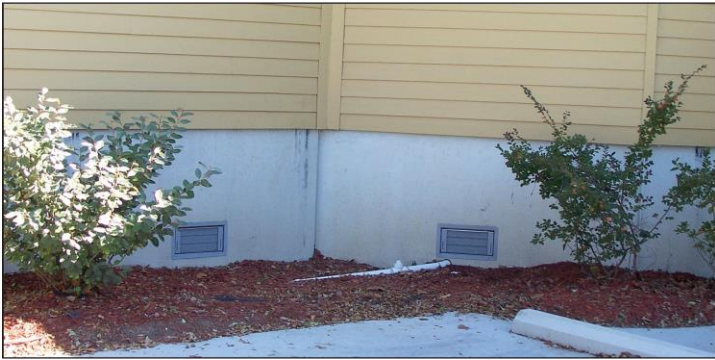
Non Residential structure retrofitted with flood
