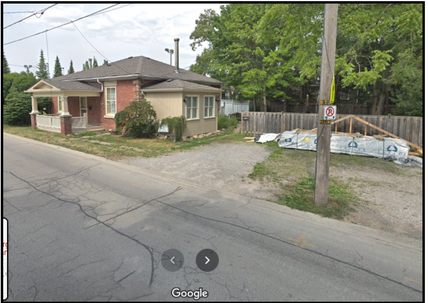
Figure 2- Photograph of the Wilson Freel House
