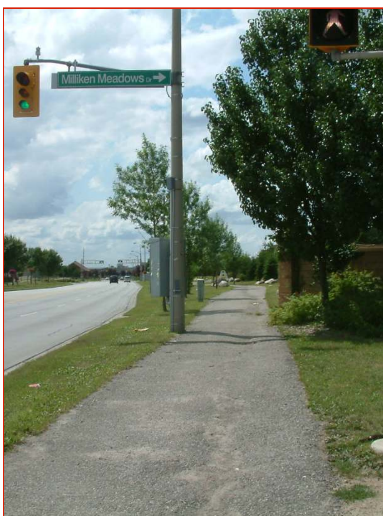
Multi-Use Boulevard Pathway - Denison Street
