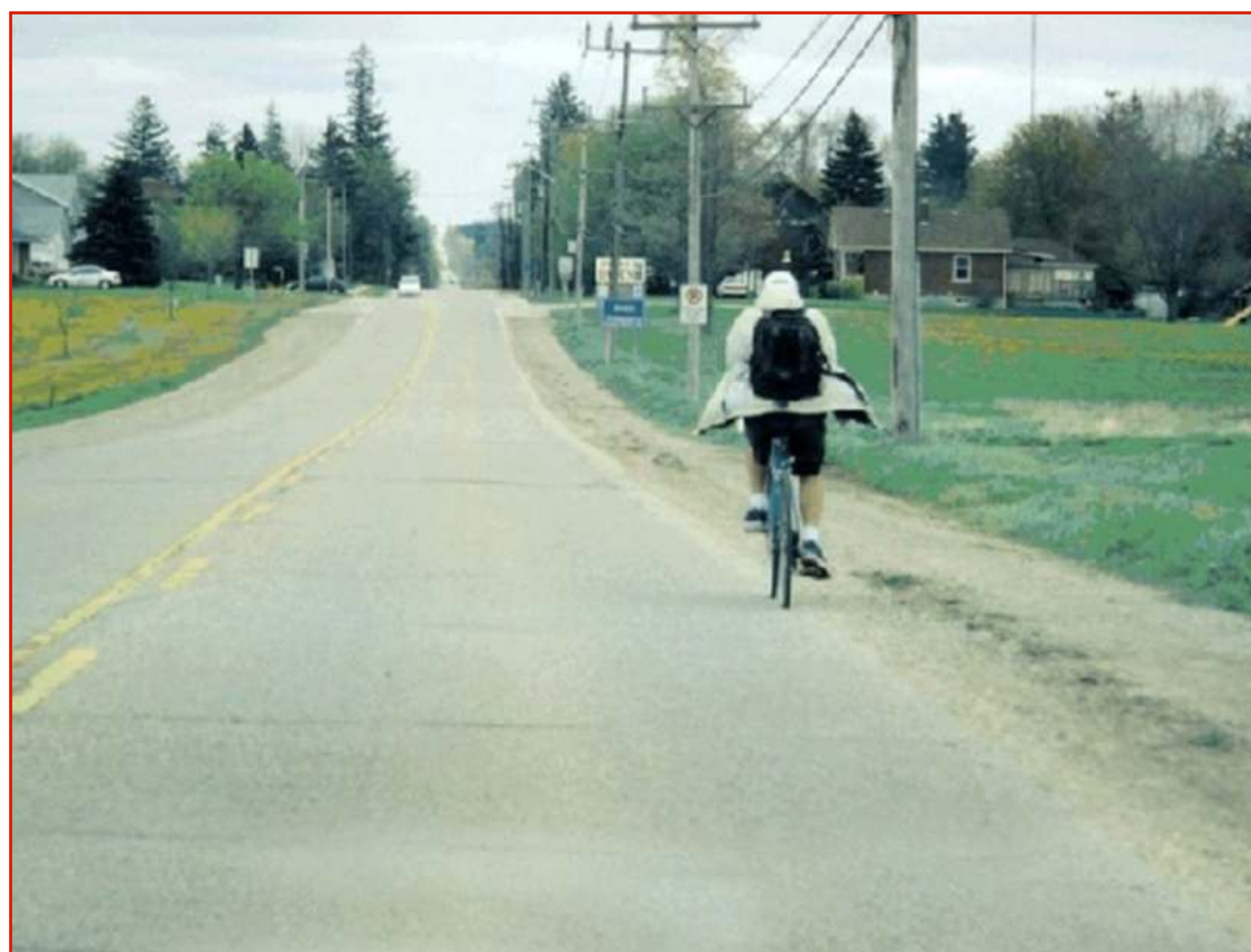
Example of a Cyclist on a Rural Regional Road with no paved shoulder
