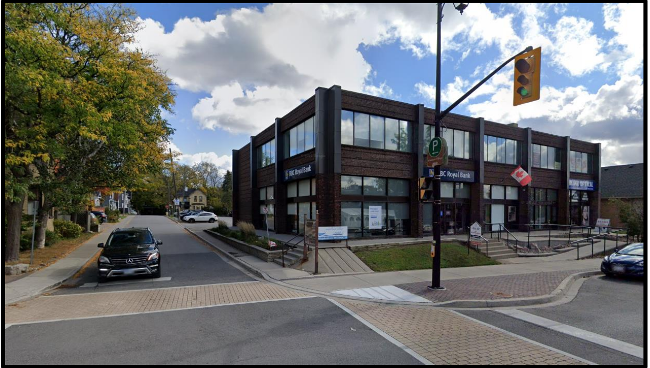
FIGURE 2- PHOTOGRAPH OF THE EXISTING BUILDING
