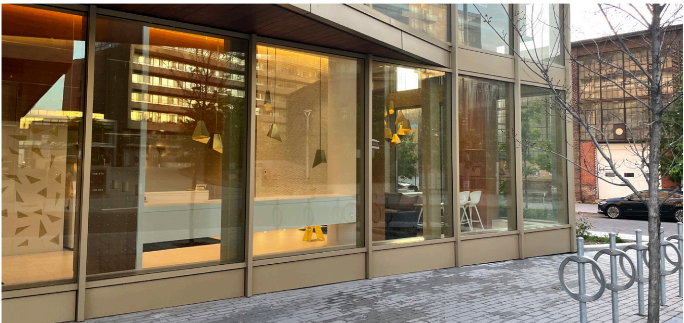
Figure 66. This lobby provides strong visual connections to the sidewalk and passenger pick-up and drop-off area with indoor seating areas.
