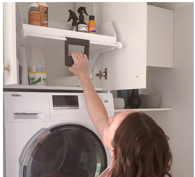
Figure 102. Pull-down shelving is a great option for older adults with limited reach as well as additional storage space for families.
