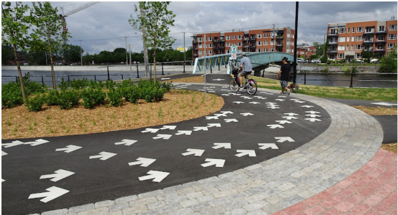
Figure 29. A cycling roundabout is playful while reducing the risk of accidents in Montreal.
