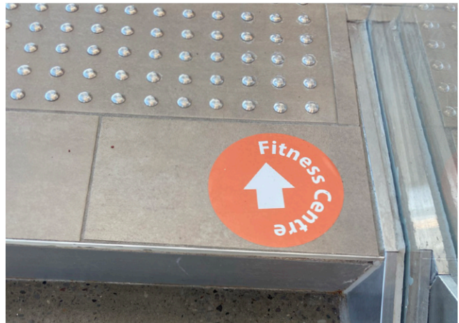
Figure 75. Tactile features at the top of a common stairway with integrated wayfinding.
