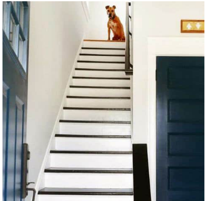
Figure 114. This straight flight of stairs shows how high contrast nosing on the steps can improve safety for some older adults with reduced eye-sight or limited depth perception.
