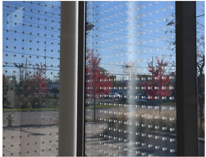
Figure 85. This bird-friendly treatment at the Markham Pan Am Centre is also helpful for retail uses with expansive glazing to reduce the risk of injuries for older adults and children.
