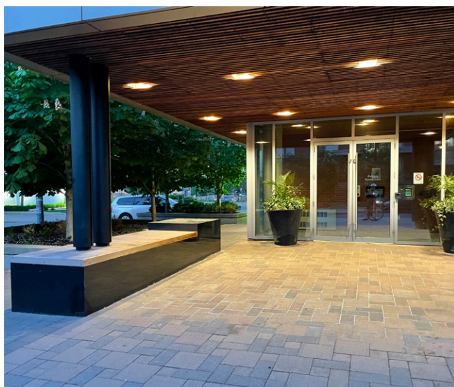
Figure 67. This building entrance is well-lit, weather protected and provides higher bench seating heights suitable for older adults.
