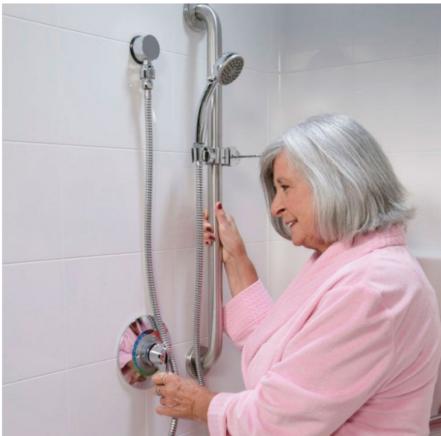
Figure 97. Handheld shower heads on grab bar sliders provide the flexibility to be useful for many types of households.
