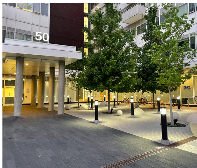
Figure 64. The site design for this development oriented the buildings to provide a landscaped forecourt and generous entry plaza.
