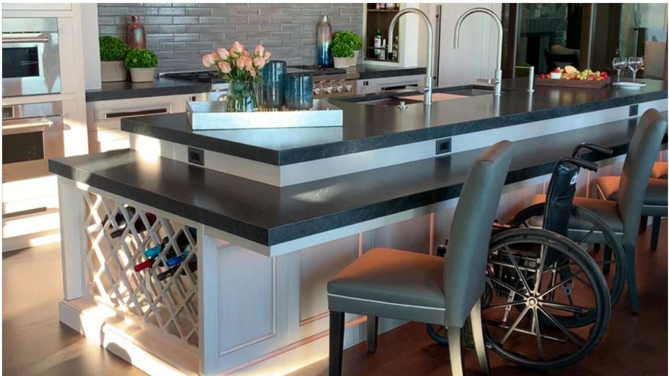
Figure 93. Multi-height countertops or kitchen islands are beneficial for older adults as mobility is reduced, but also practically provides added flexibility and additional seating for other households.
