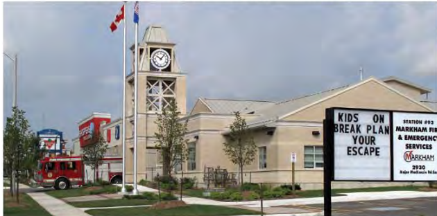
Fire Station 93: 2930 Major Mackenzie Dr. East (Built 2010)
