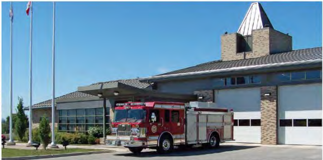
Fire Station 92: 10 Riviera Drive (Built 2003)
