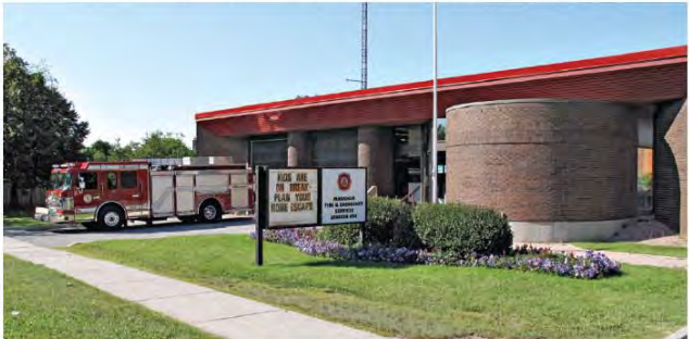
Fire Station 94: 7300 Birchmount Road (Built 1980)
