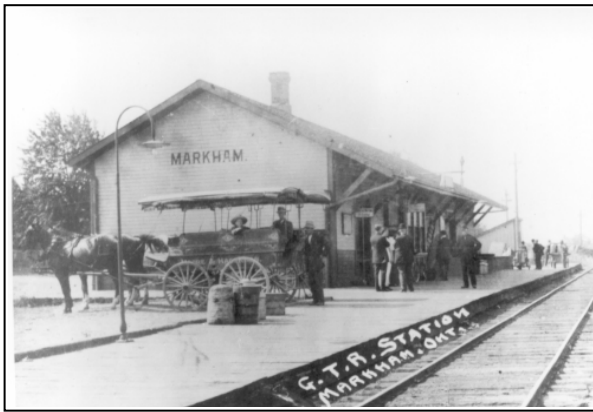
Markham Village Train Station, c.1900
