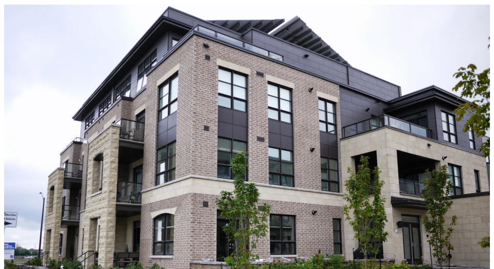
Solar panels integrated into building design
