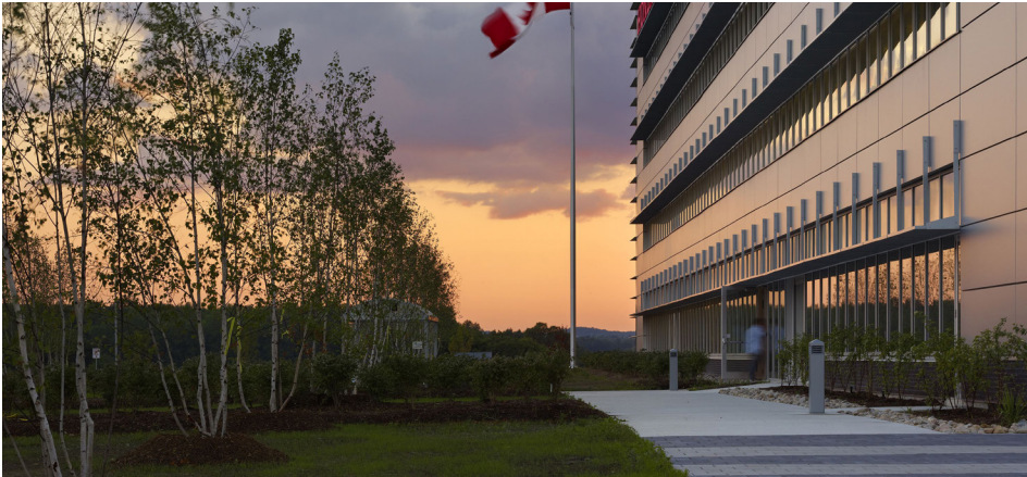
Outdoor amenity areas and landscaped walkways add interest to office buildings
