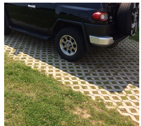
Pervious pavers in parking lot
