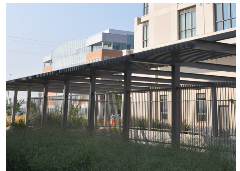
Entrance to underground garage screened using decorative walls, trellis and landscaping
