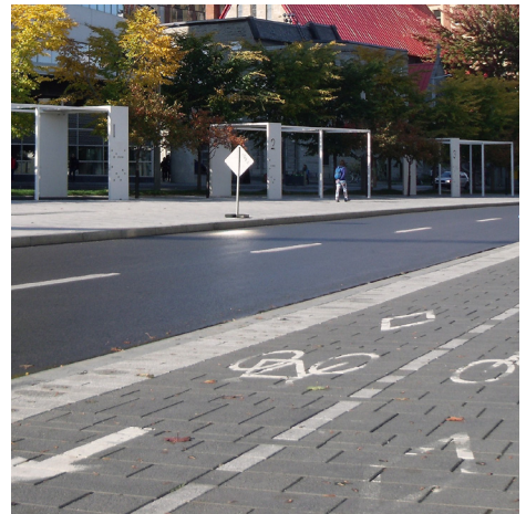
Clearly demarcated zones for pedestrians, cyclists, and motorists enhance safety
