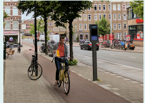
Raised and separated cycle tracks provide dedicated cycling facility on boulevards
