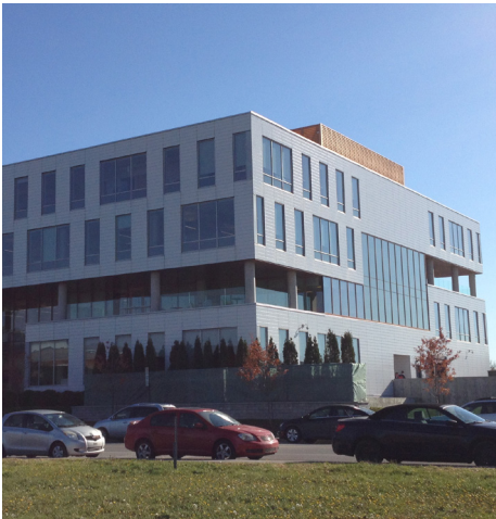
Well-screened rooftop mechanical equipment
