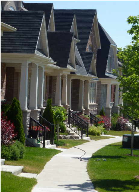
Walkways connecting entrances to sidewalk
