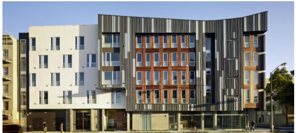
Materials and colours are used to break down the mass of larger buildings
