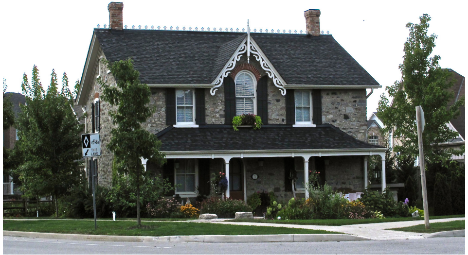
Heritage structure located on a corner lot, with strong relationship between front door and the street
