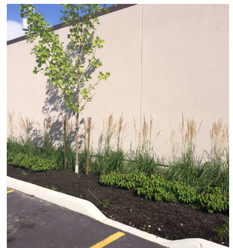
Landscape area in surface parking lot used as LID feature for stormwater management
