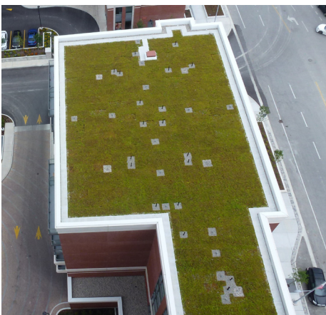
Green roof to reduce environmental load
