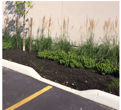
Landscape area in surface parking lot used as LID feature for stormwater management
