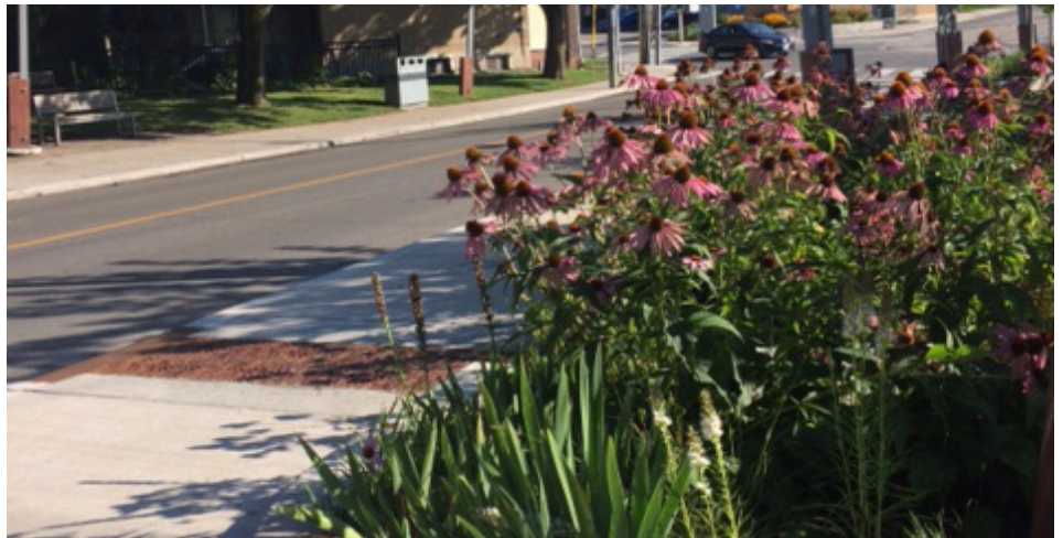
Rain gardens minimize stormwater runoff and provide additional visual amenities within the public realm
