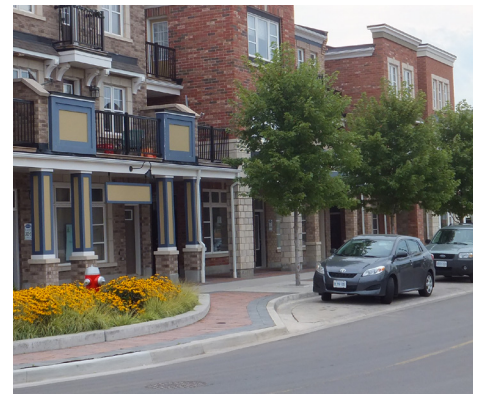
Main street with enhanced streetscape and on-street parking
