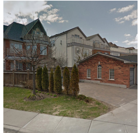
Adequately screened service area with dedicated areas for waste storage
