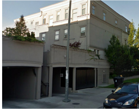
Private amenity area above the garage
