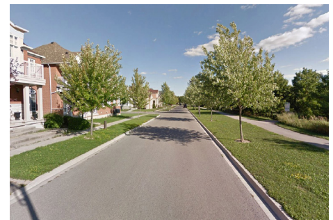
Single loaded road along the Greenway System
