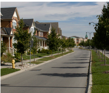
Building height, massing and planting providing street enclosure
