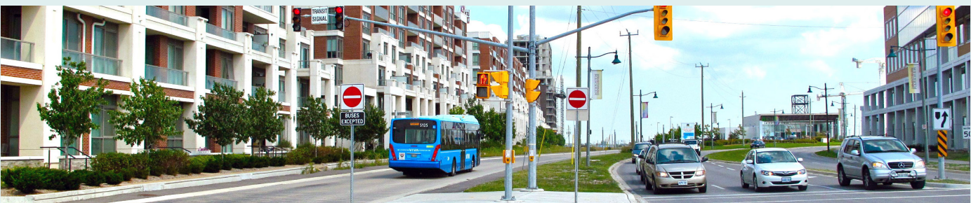
Dedicated bus lanes ensure that public transportation remains an efficient and viable option for commuters with choices
