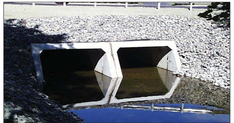
Twin Existing Culverts Under Roads/Parking Lots
