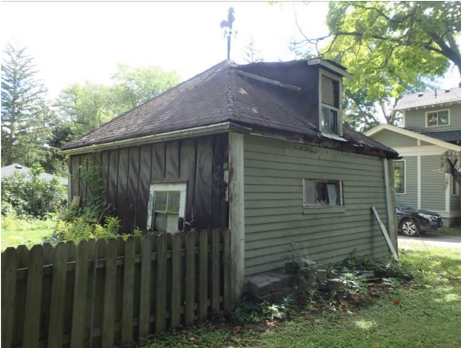
Existing garage, 2020 (Heritage Section Photo Collection)
