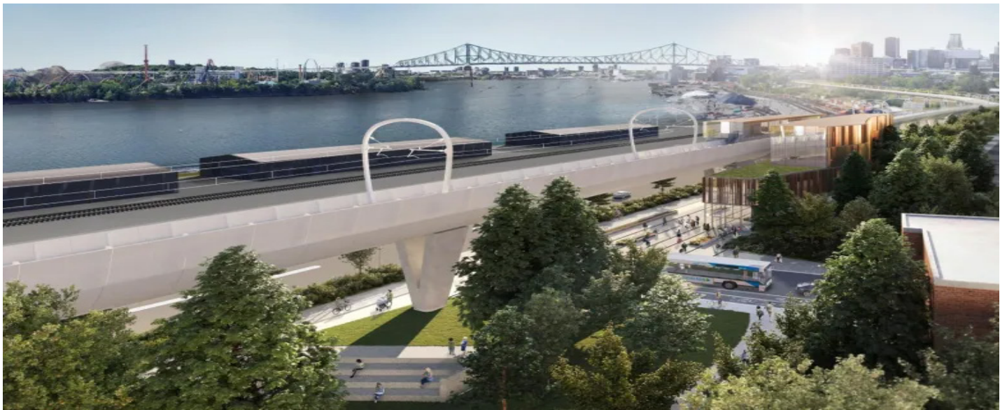
Figure 11. New Elevated Track Designs for Montreal's REM de l'Est Address Concerns - East REM2
