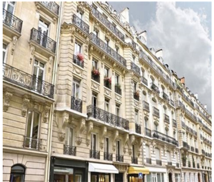
Figure 8. Parisian Building - Paris, France
