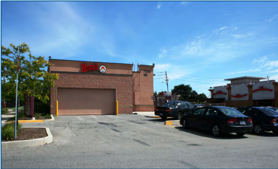
Figure 4.9a: Wendy's restaurant on Steeles & Woodbine - photograph demonstrates how to appropriately situate and enclose garbage areas at the rear, and within the building.
