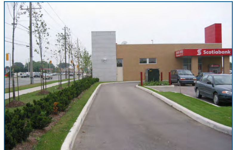
Figure 4.8b: This Scotia Bank on the Queensway & Islington in Toronto illustrates an adequate landscaped screen between the road and the stacking lane.
