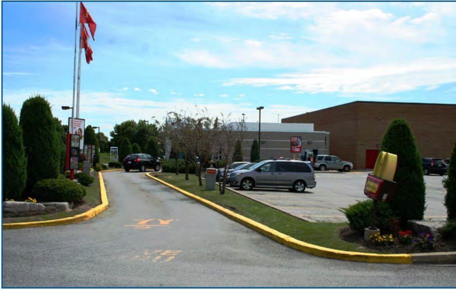
Figure 4.5d: McDonald's on Kennedy Road & Lee Avenue - provides adequate landscaping and clearly distinguishes stacking from parking areas.
