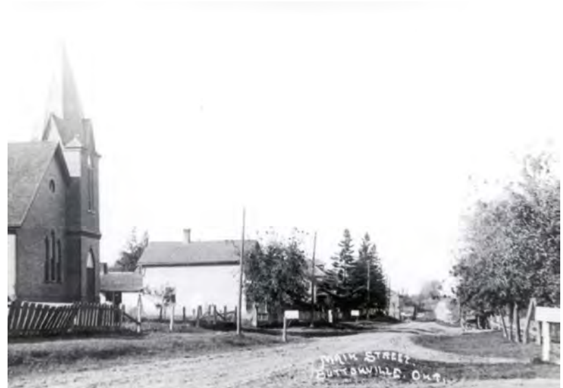
Buttonville -1909. View north on Woodbine Avenue. Only some foundations remain of the Lutheran Church on the left. Casella #24
