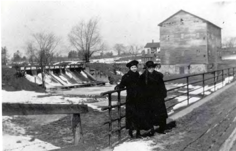
The Buttonville Heritage Conservation District boundaries focus on the core of the hamlet that grew up around the local milling industries. Casella #22
