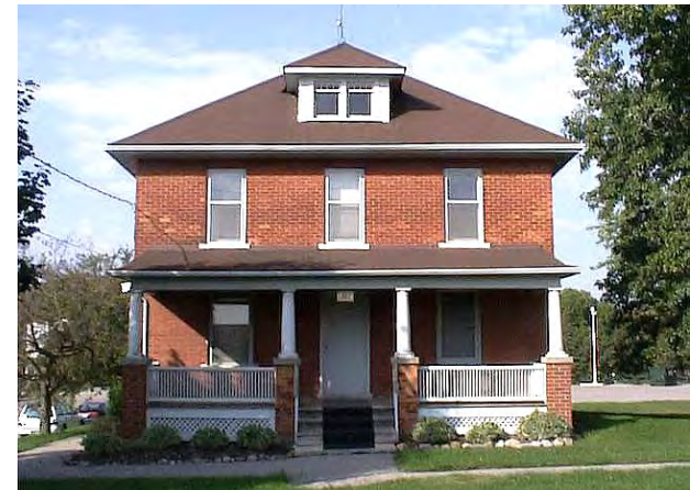
The Mill House at 9064 Woodbine Avenue was originally a 1-1/2 storey Georgian house, associated with the Venice Mill.
