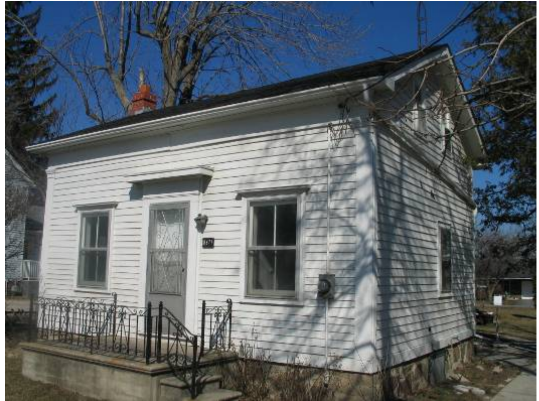
The Button House, c.1850, at 8977 Woodbine Avenue, is a fine example of a vernacular house with Classic Revival details. Note the cornices over the front door and windows, and the substantial corner pilasters.
