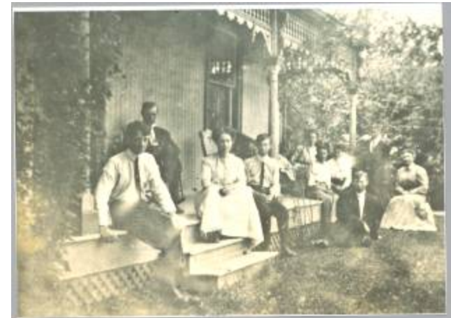
Late 19 th century veranda on the Hood Farmhouse. Casella Historical Collection #43
